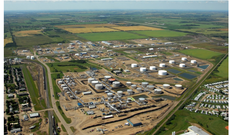
Asphalt Refinery and Pipeline Terminal
