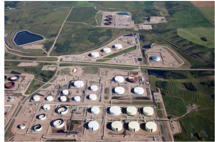
Hardisty Pipeline Terminal
