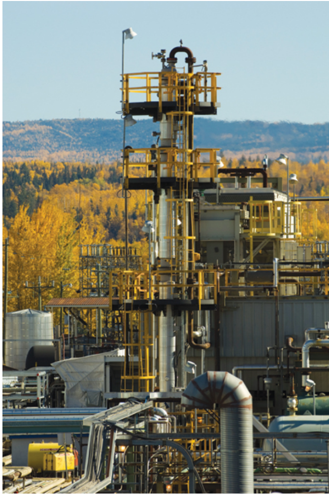
Prince George Refinery
