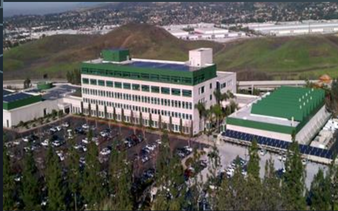
SCAQMD Headquarters Diamond Bar, California
