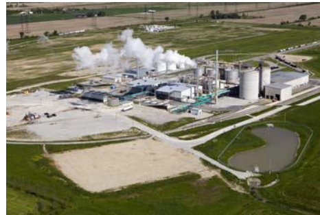
St. Clair Ethanol Plant
